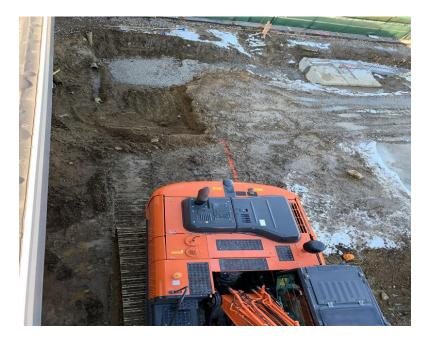
The renovation work in the areas where the new main office and STEAM bar classrooms will be located continues forward. Footings were dug in the STEAM classrooms for the columns that will support the roof and the new main corridor.
